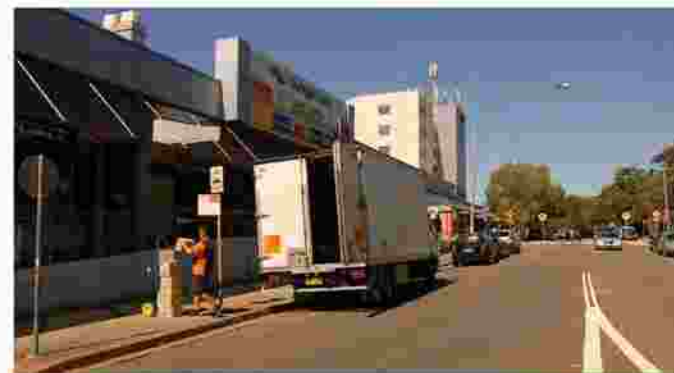
Existing Bungan Street South
